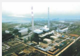
Thermal Power Projects
